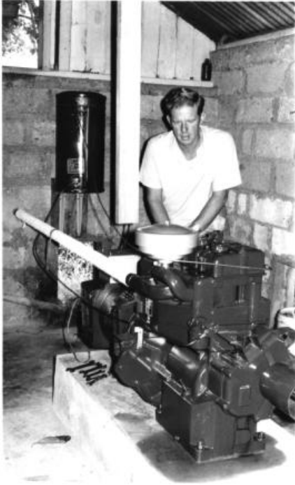
Fr Alan Finn fixing the generator
